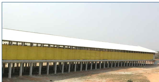
Figure 4. Lowering the curtain at the top creates better ventilation.
